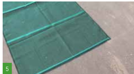
5 Lay a Group 2 tarpaulin with the openings facing up. Put the PVC pipe in the bottom hem, with the sleeve on the left.
