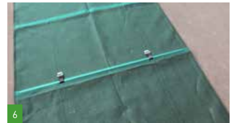
6 Put the steel tube in the right hem and place the buckles at the openings. Do this for all the tarpaulins in group 2.
