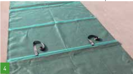
4 Put the steel tube in the right hem; estimate the pit height. Put the tension straps around the tube at the openings. Do this for all the tarpaulins in group 1.
