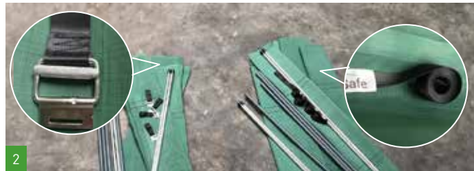
2 Split the material into 2 groups. Group 1: half of the tarpaulins, PVC and steel tubes and all tensioning straps. This is for the left silo wall, seen from the pit entrance. Group 2: the other half of the tarpaulins, PVC and steel tubes and all buckles. This is for the right silo wall, seen from the pit entrance.
