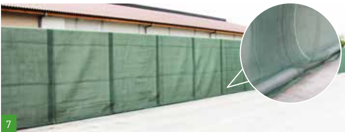
7 Lay the tarpaulins from group 1 over the left wall (seen from pit entrance), with the sleeve facing forward. Slide the tubes together. Always make sure that the rear tarpaulin overlaps the tarpaulin facing it. Do the same on the right side with the tarpaulins from group 2.
